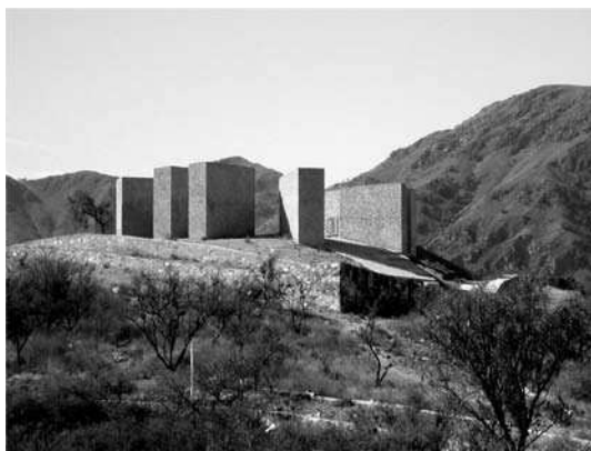
Figura 1. Plaza del Cerro. Vista General. Plaza of the Hill. General sight.
